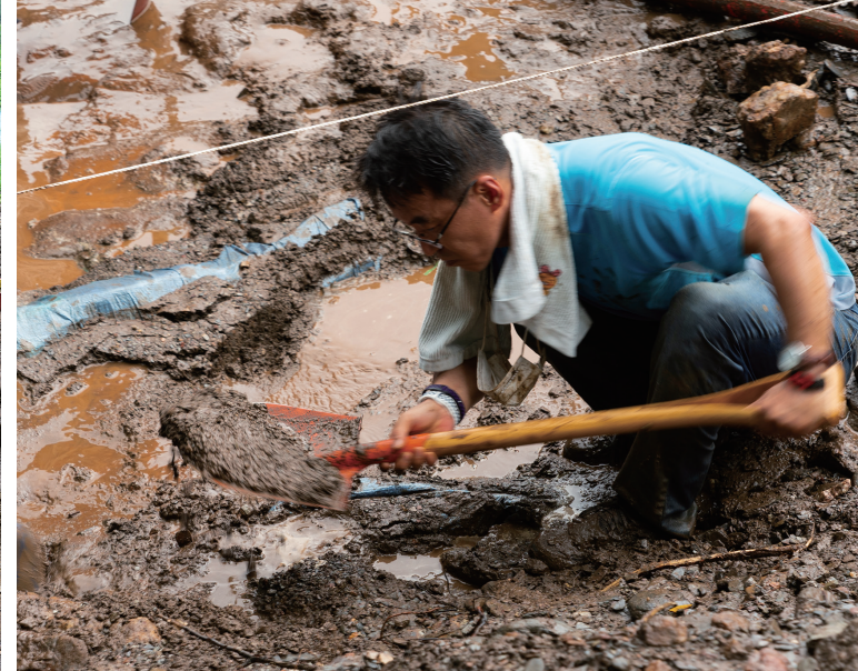
An excavation crew member digging up a drainage ditch in the sudden torrential rain
